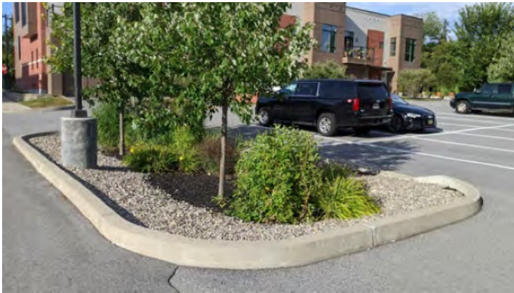
Figure 22. Stormwater retention in a parking island.
