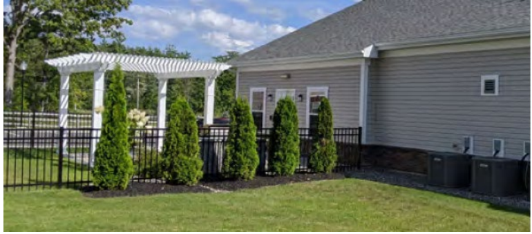
Figure 25. Screening of mechanical equipment.
