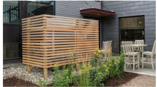
Figure 28. Screening of mechanical equipment.
