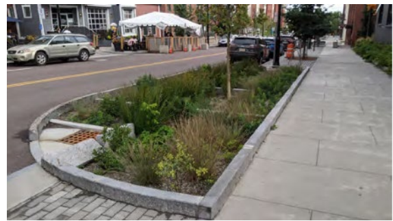
Figure 21. Stormwater retention with rain garden.
