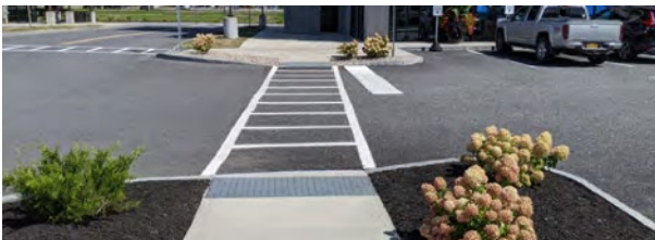
Figure 17 Internal parking lot crosswalk.
