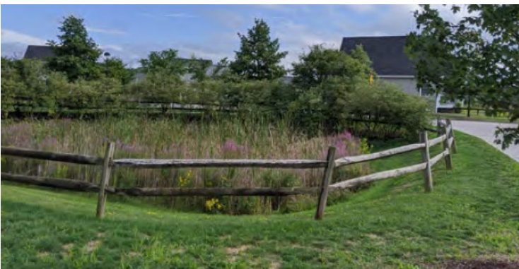
Figure 23. Stormwater retention pond in a housing development designed to look like a natural pond.
